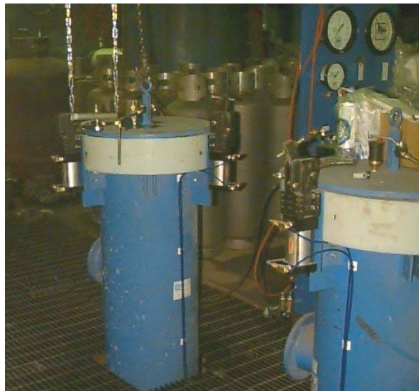
Figure A-2. Water-filled jacket (test chamber) in which hydrostatic and burst testing were performed.
